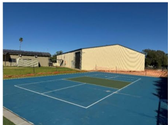
Figure 4 Outdoor Pickleball Court at Youth and Community Centre (grandstand not yet installed)
