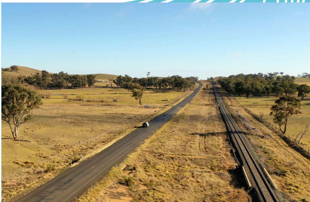
Aerial of regional road and rail track near Dubbo
