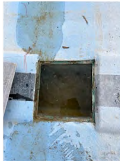
Deep culvert in main pool, unknown depth
