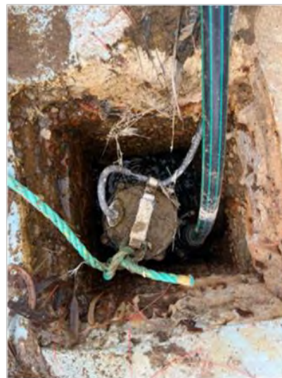
Deteriorated pump
