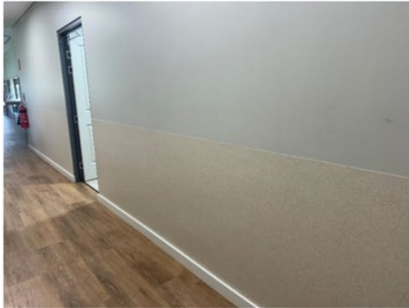
Figure 1 Protective wall vinyl installed throughout the Youth and Community Centre.
