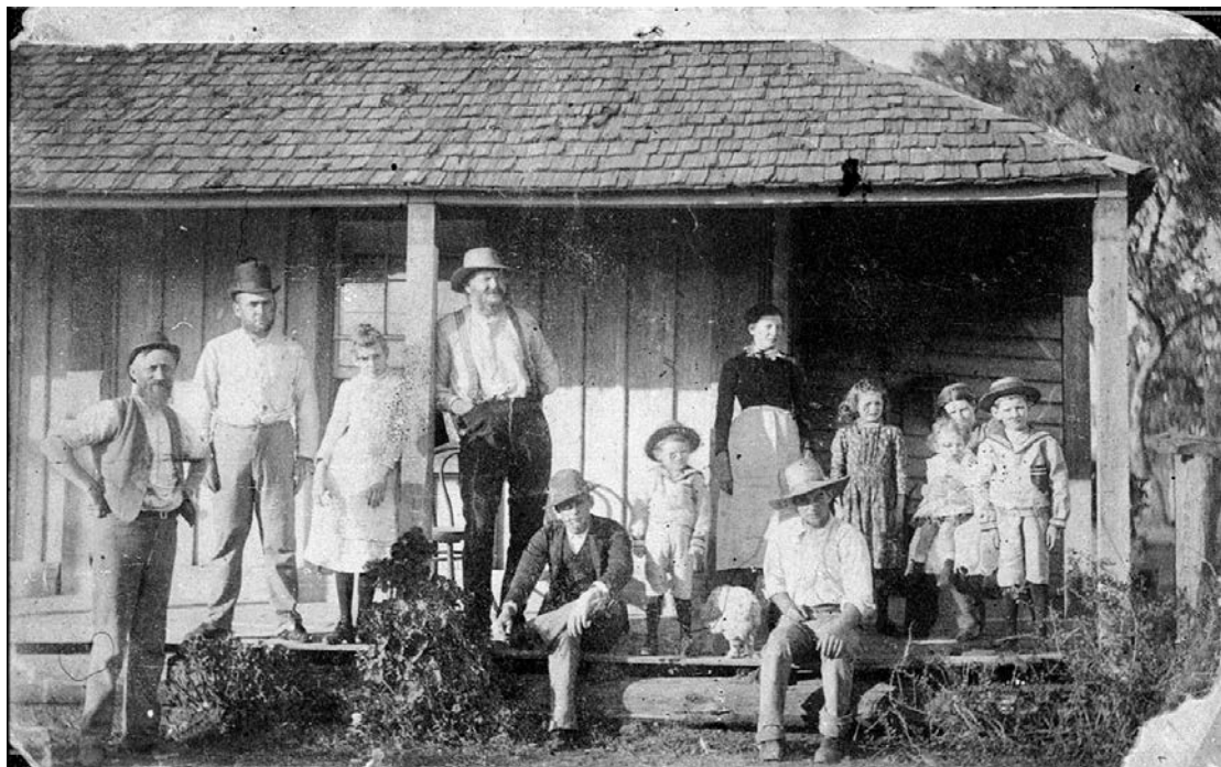
Figure 16 This photo of the Buddabaddah Hotel in November 1890 shows the slab and shingle construction used in early housing in rural areas. Source: ML, At Work and Play 03524
