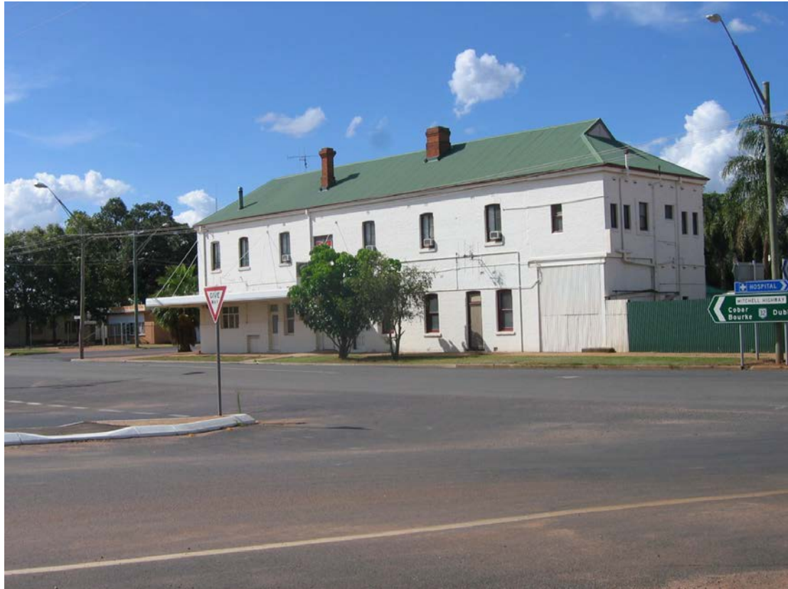
Figure 21 The former Commercial Hotel, Nymagee Street, Nyngan.
